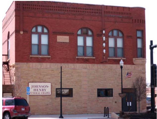
The corner turret that once predominantly marked the intersection of 3rd Street and Main Avenue was removed and capped due to significant damage sustained from a high-wind storm during the 1930’s. In 1954, the front of the building was covered with stone, the doors were replaced and a garage was added to the rear of the building.
