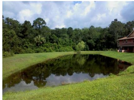
**Detention pond** is a normally dry reservoir where stormwater collects and is temporarily stored. The water slowly drains into a receiving channel usually within 24 hours.
