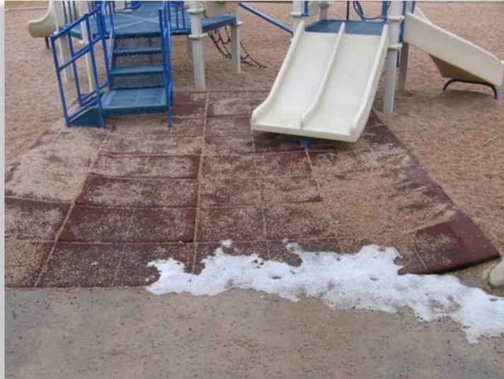
Tile surface has curling edges, gaps, and excessive cross slope. Loose fill (pea gravel) contaminates the tile surface.
