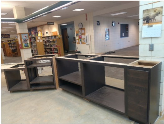
New carpet and circulation desk install
